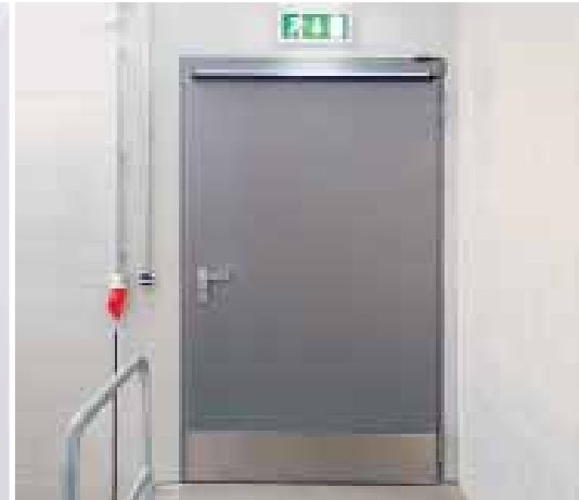
T90-1 type N19 Door with thick rebate
